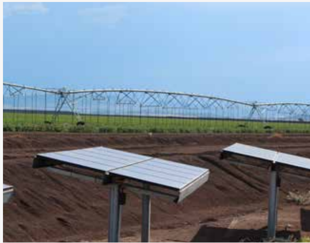
FIGURE 2: Solar array mounted over an irrigation delivery channel under a space-restricted scenario
