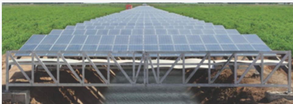
FIGURE 2: Solar array mounted over an irrigation delivery channel under a space-restricted scenario
