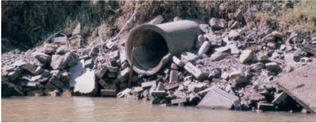
Stormwater pipe carrying stormwater runoff directly into the river and reducing water quality. Photo Guy Roth.
